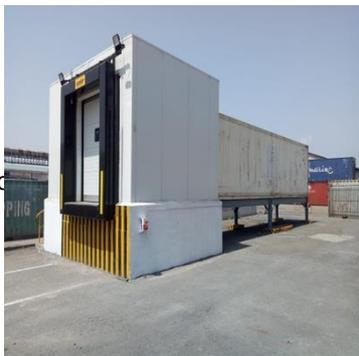
The infrastructure includes a 40 feet air tight Central Refrigerated Compartment with adequate safety controls. The Reefer container under inspection/ reworking can be directly connected to the Compartment on trailer and necessary work can be done. This facility would be made available for customers during this reefer season. This is aligned towards our motto of "CUSTOMER FIRST".
