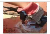
MT inspection after crack removed by grinding
