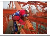
Crack repaired by welding repairing in progress
