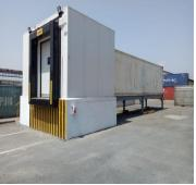
The infrastructure includes a 40 feet air tight Central Refrigerated Compartment with adequate safety controls. The Reefer container under inspection/ reworking can be directly connected to the Compartment on trailer and necessary work can be done. This facility would be made available for customers during this reefer season. This is aligned towards our motto of "CUSTOMER FIRST".
